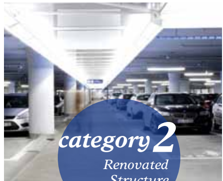
Stachus car park, Munich (Contipark)
